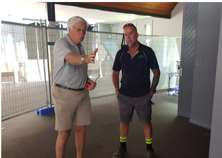
John gives Sean some building instructions as the GA refurbishment begins
